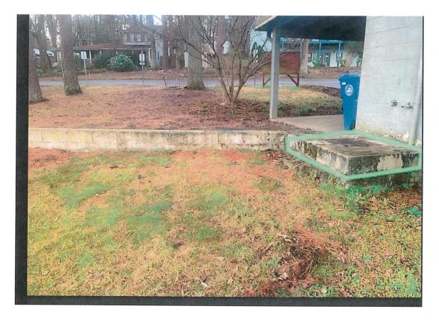
New concrete will be broom finished will drainage fall
